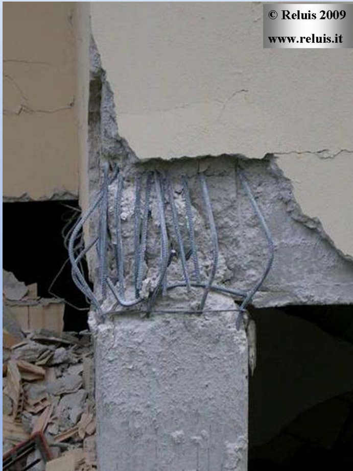
No stirrups in the joint
