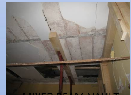
MIXED BEAM-VAULT FLOOR SLAB
