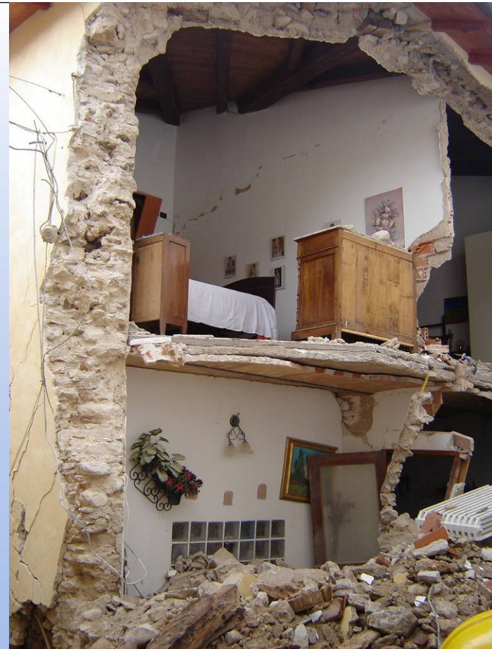
Paganica: insertion of a deep r.c. slab
