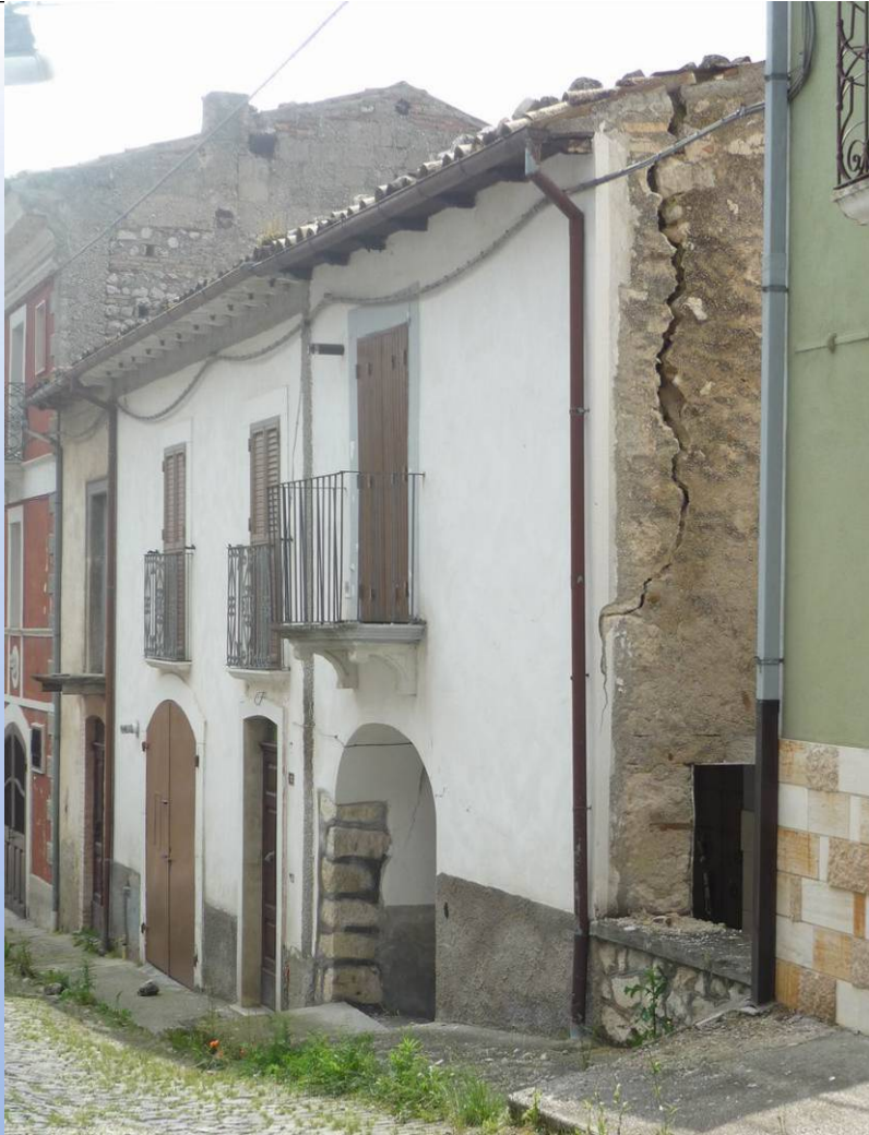
Castelnuovo: poor connection between masonry walls.
