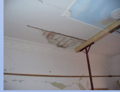
MIXED BEAM-VAULT FLOOR SLAB
