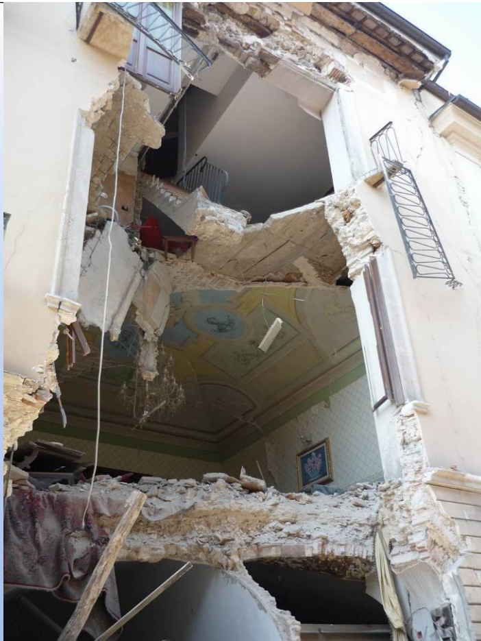
L'Aquila: at second floor it was inserted a r.c. stair.
