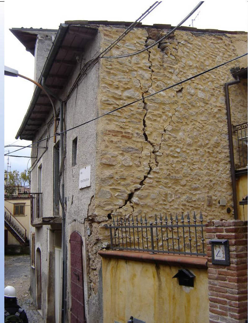
Paganica: overturning crack involving a portion of masonry wall.
