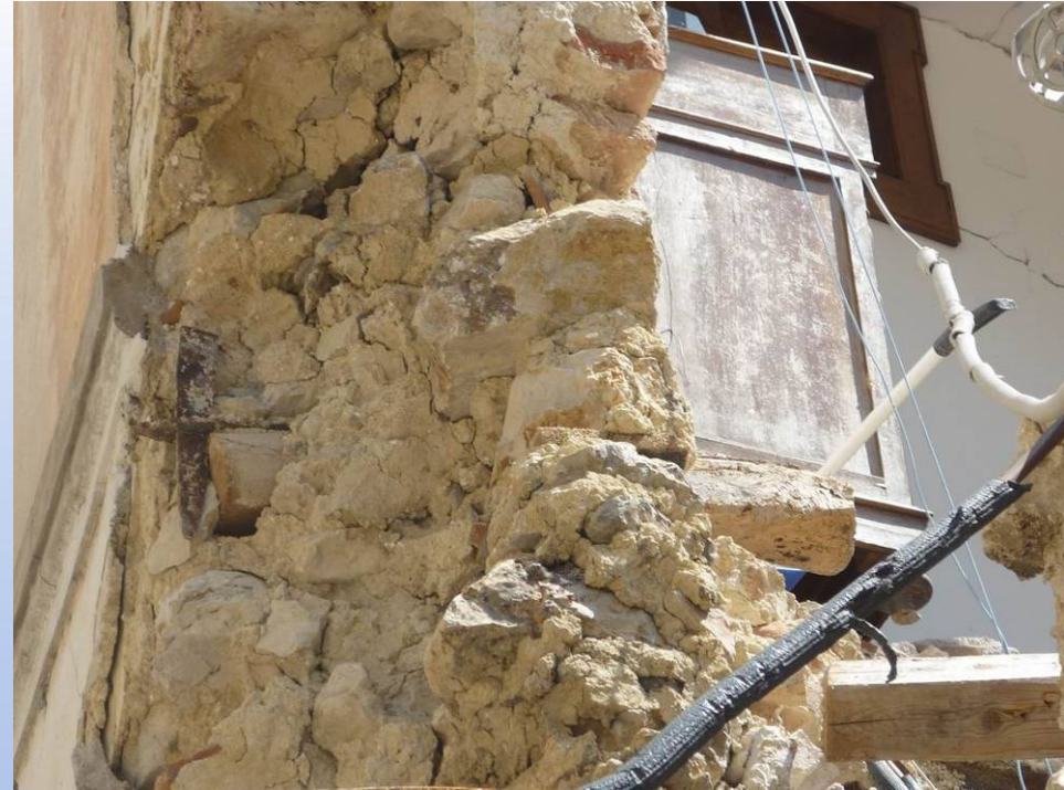
Villa Sant'Angelo: alteration of the original structural configuration: wooden tie, originally well connected to the external wall by means of an iron device, has been cut during an heavy refurbishment
