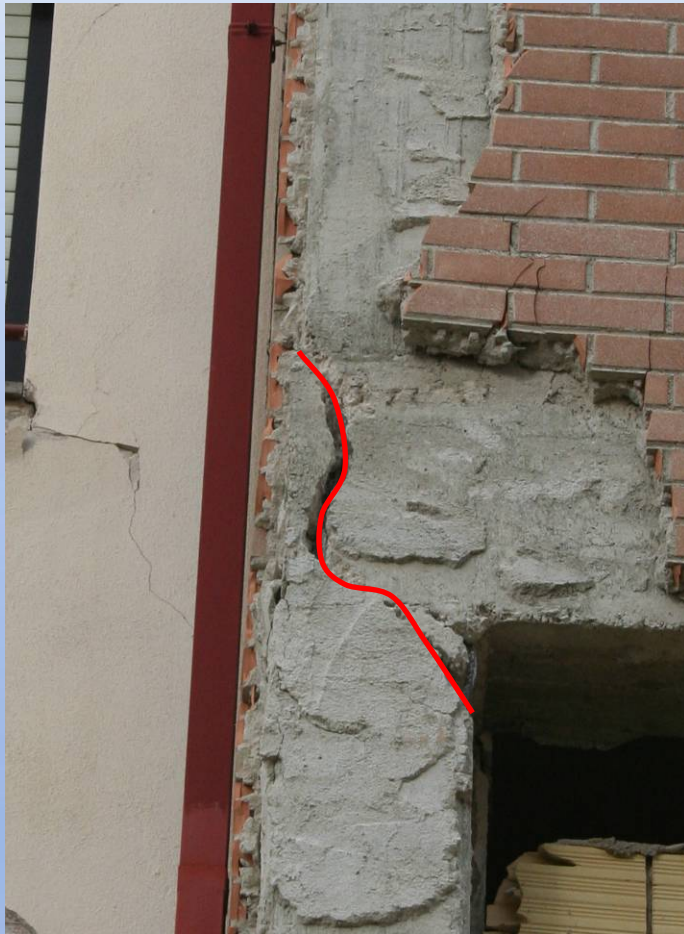
Lack of stirrups in the joint
