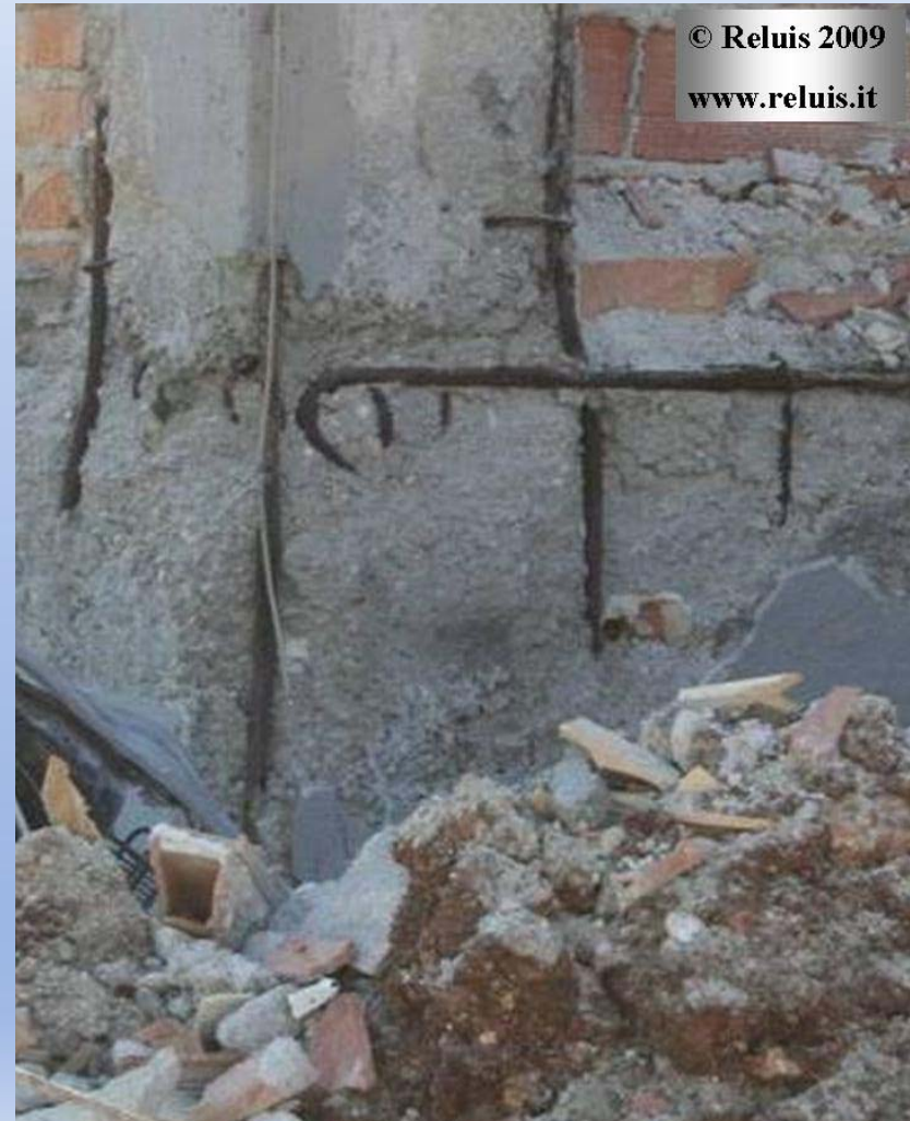
Poor concrete quality
