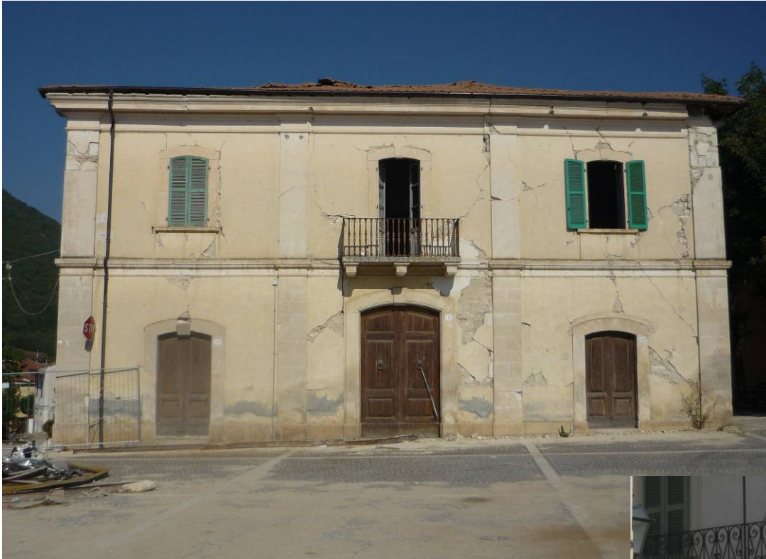
Villa Sant'Angelo: in-plane shear cracks on the whole facade wall.
