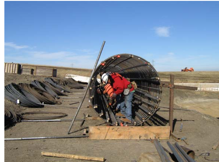
Iron Workers making rebar cage for Bent 4R CIDH/COLUMN.
