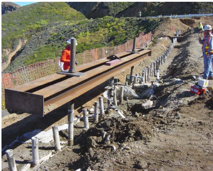
Micropile load test performed by Foundation Testing Branch.
