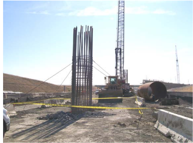
Guy wire on a short column.
