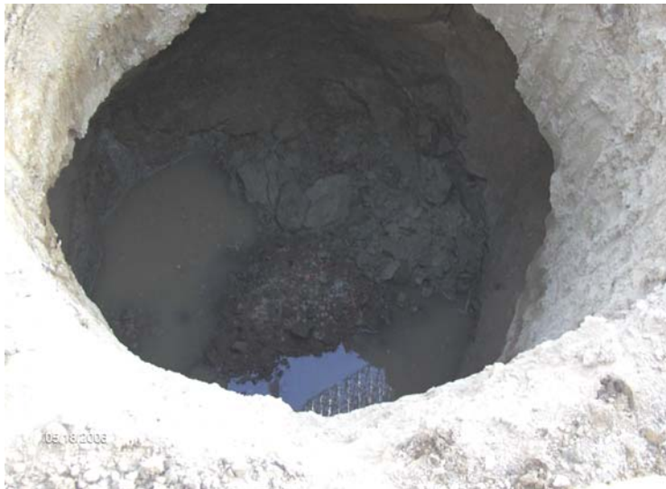
Cave-in at Bent 3 of the 580/205 Separation Bridge.
