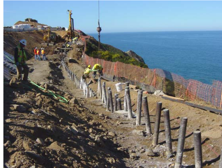
Foreground: battered micropiles, facing south. Background: Pacific Ocean.
