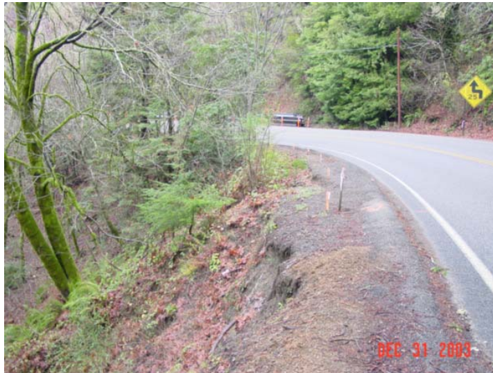
“Before”. Facing east. Survey stakes placed. Slope is eroding (on the left). 12/31/03
