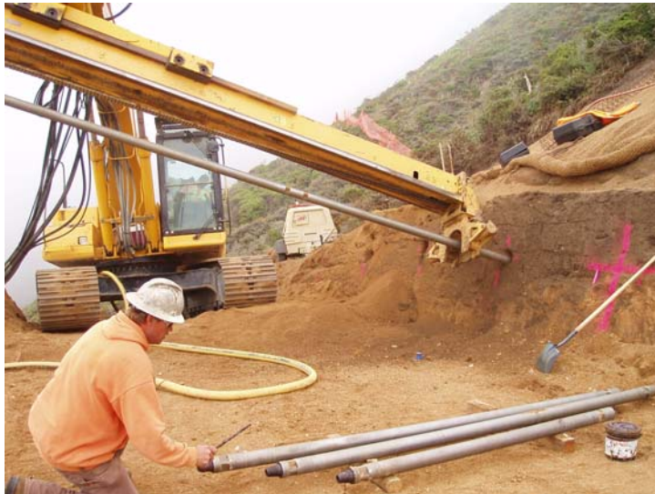
Drilltech begins drilling at Wall #2. 8/04/05
