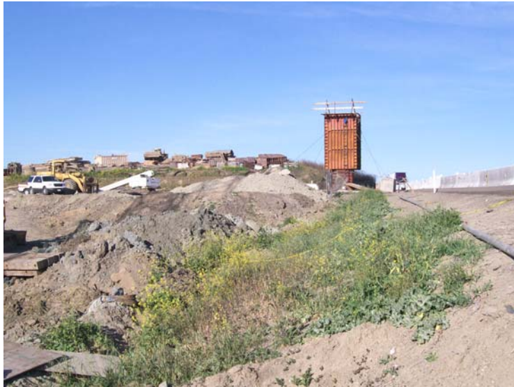
Guy wire placed on the column forms.
