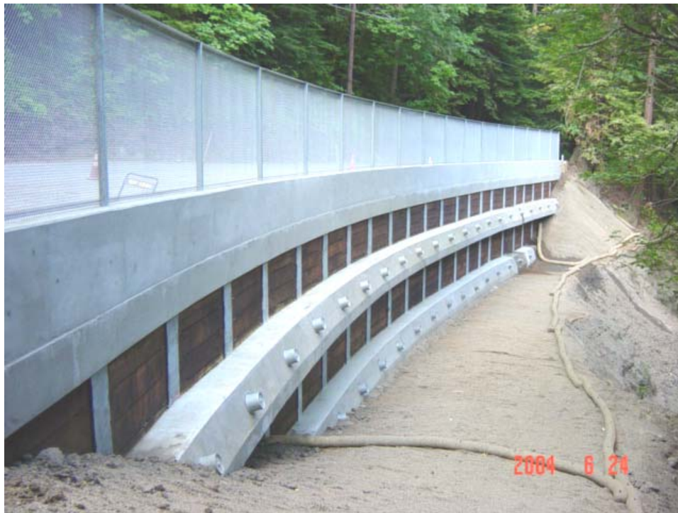
Soldier Pile Wall with Tieback Anchors within two concrete walers. Date: June 2004. Fiber rolls placed along slope for erosion control. Photo by D. Dait, P.E., Sr Br Engr
