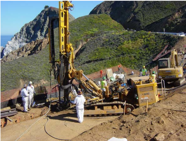
Left: Crawler mounted drill rig w/hydraulic rotary percussive head; hose grout hose on left. Right: excavator.
