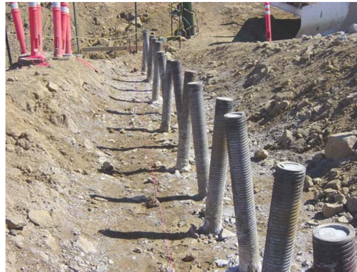
Battered micropiles. Facing north.
