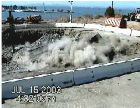
Photo 1. Pier W2. Before detonation. Blasting mats on top.
