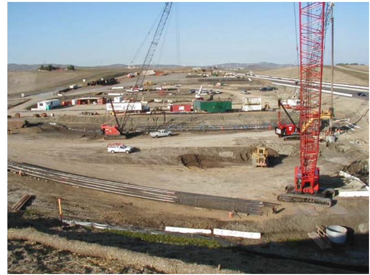
Bent 7 cage; Bent 6 drilling.
