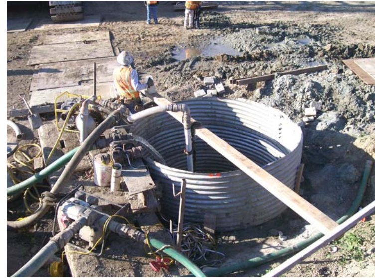
Contractor placing SlurryPro CDP with CMP casing used to prevent cave-in @ Bent 5 of the 580/205
