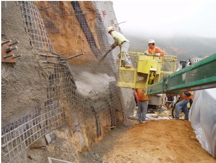
Drilltech workers shotcreting at Wall #1. 8/04/05
