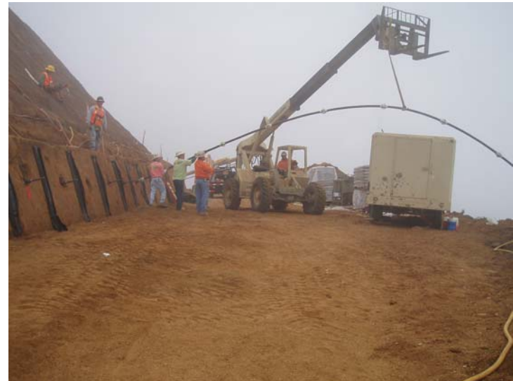
Drilltech installing soil nails with forklift at top row of Wall #2. 8/05/05
