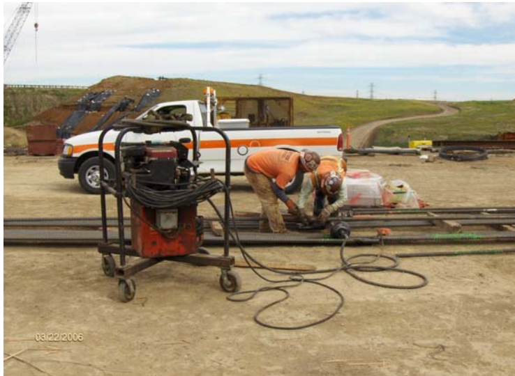
Rebar coupler splice equipment in use.
