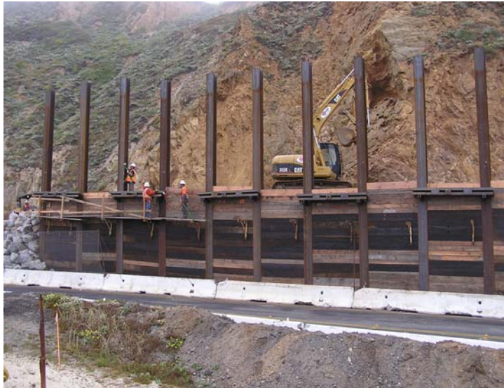
GNB installing tieback walers at temporary shoring wall at Wall #1. 6/28/05
