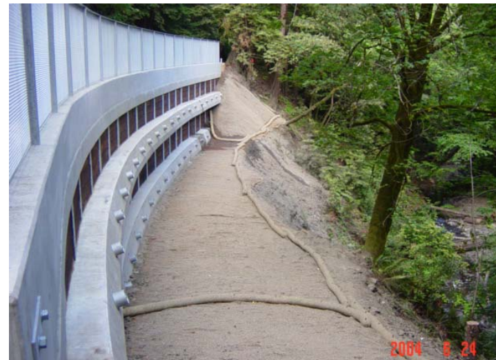
“After”. Facing west. Wall is complete. Two rows of concrete walers (with tieback anchors). Creek on the right. 6/24/04
