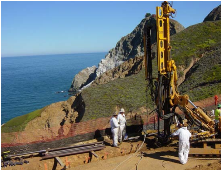
Drilling/installing micropiles. Pacific Ocean in the background.
