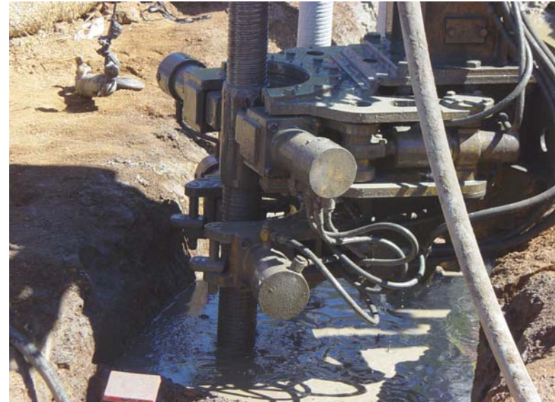
Drilling and flushing.
