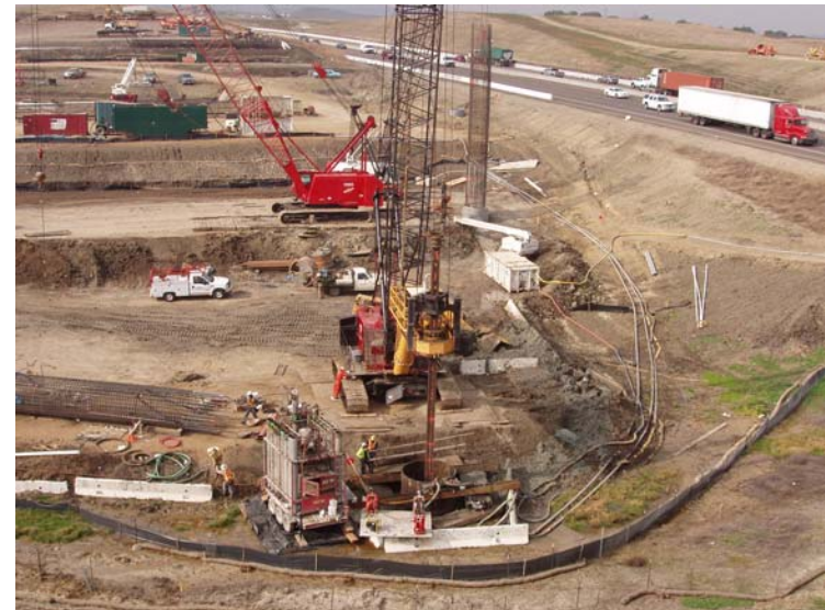
Drilling at Bent 7 with Steel casing to prevent cave-in.
