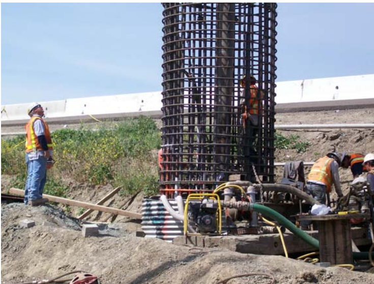
CIDH pour with tremie tube in the middle of the pile and slurry is being pump back to the tank.
