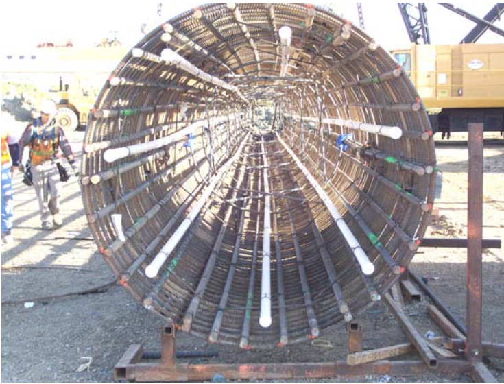
Bent 5: 180-ft long rebar cage with 3" gamma gamma PVC inspection tubes installed.
