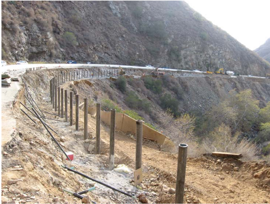
Micropile (NPS 8-XX Strong Steel Pipe) in a 300-mm dia drilled hole. On the ground - Sections of Rock Anchors to be installed later. Date: 2007
