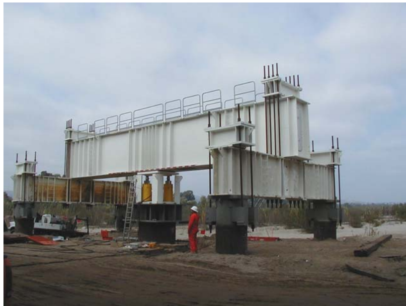
FIGURE 8-1 Static pile load test (five-pile array)
