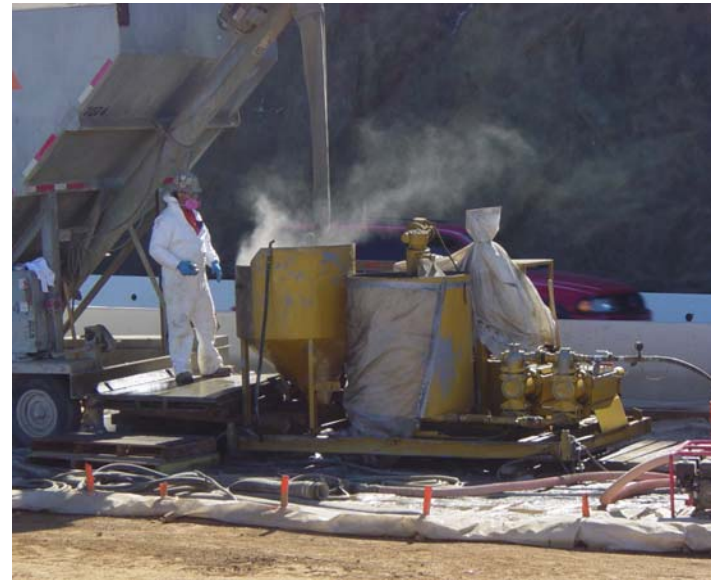
Grout mixer. Grout is pumped to the micropile drill rig.
