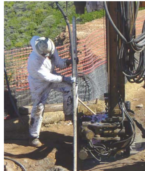
Checking top of pile elevation with a laser level (grout hose is blocking view of the survey rod).
