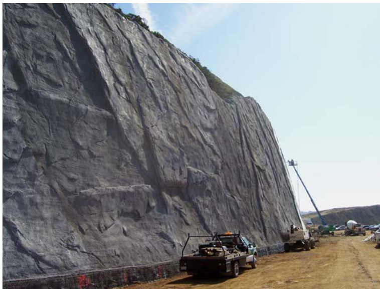
Retaining Wall #2. Shotcrete sculpting at northern end of wall.
