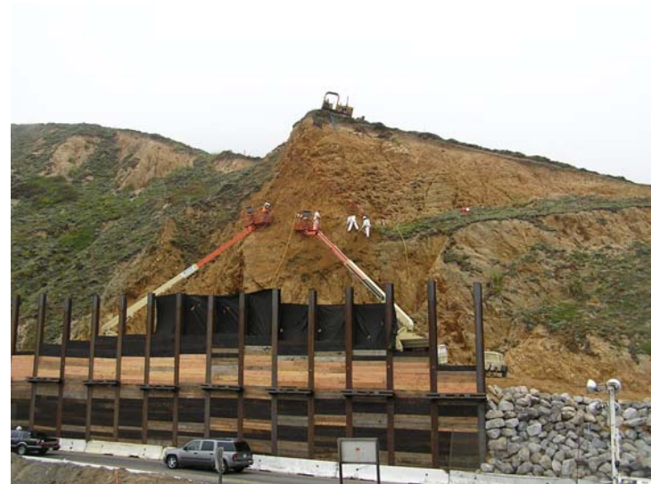
GNB begins hand excavation at Wall #1. 7/01/05
