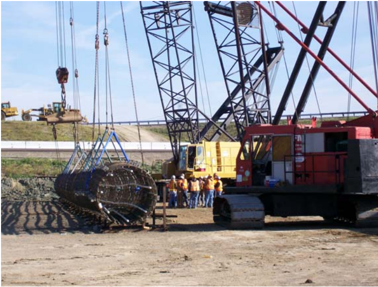
Critical lift safety meeting held just before the cage lift.
