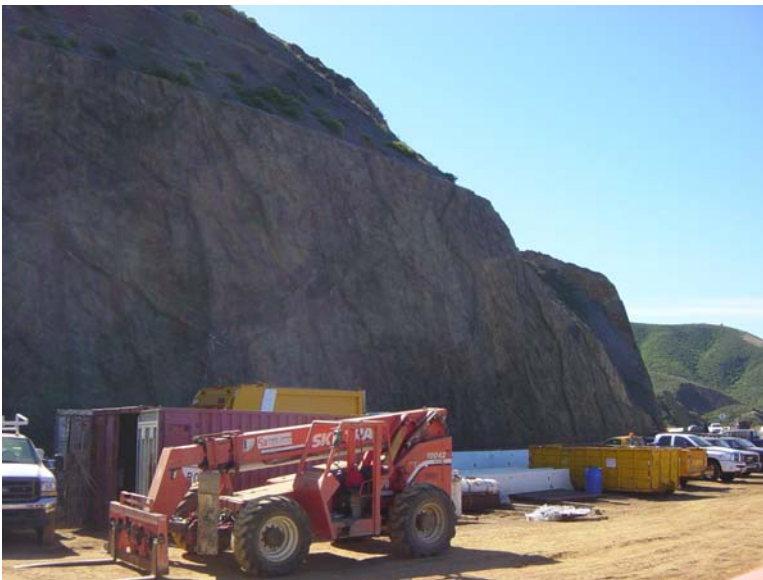
Forklift. Background: South Rock Cut Retaining Wall (soil nail wall with sculptured face)
