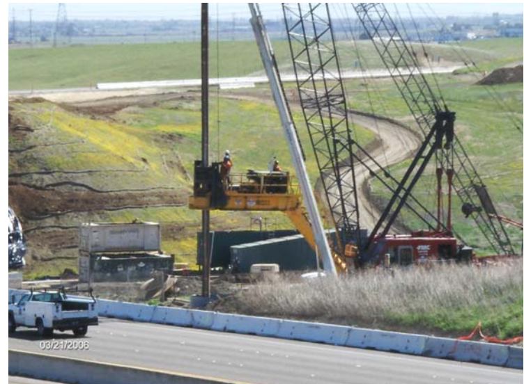
Drilling at Bent 5.
