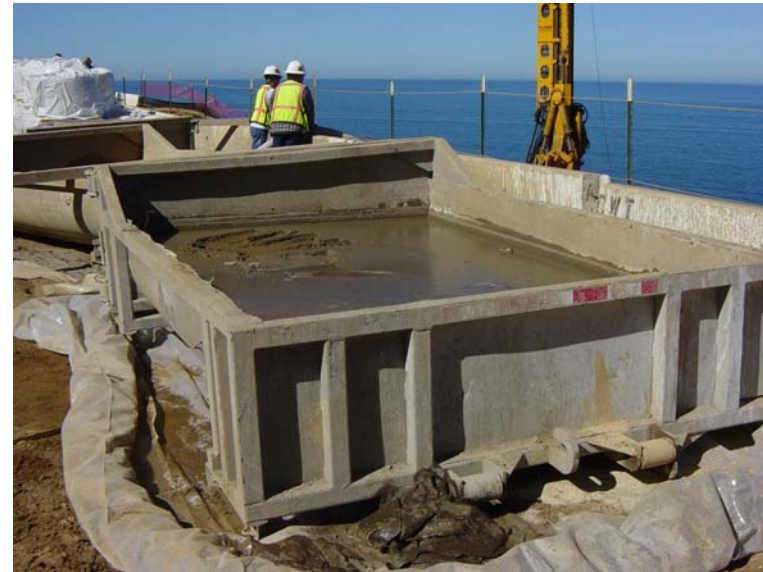
SWPPP: grout settlement container / concrete washout container.
