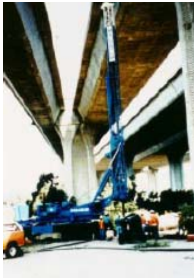
FIGURE 6-13 Drill rig – truck mounted
