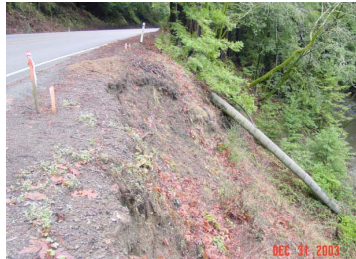
“Before”. Facing west. Survey stakes placed. Slope is eroding. Existing drainage pipe and creek on right.
