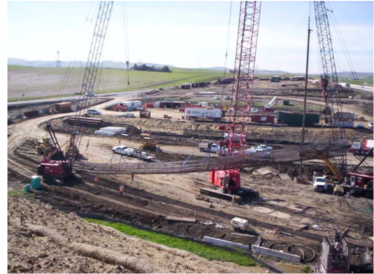
Two cranes; Bent 7 – Cage 20 pick.
