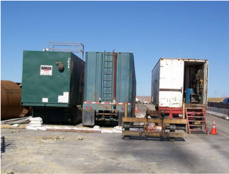
Slurry storage and setting tanks.
