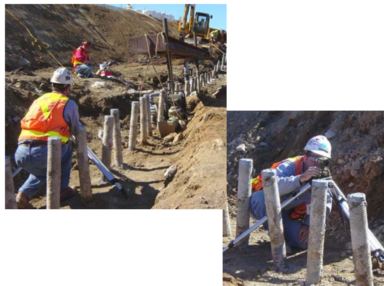
Recording measurements using auto-level.
