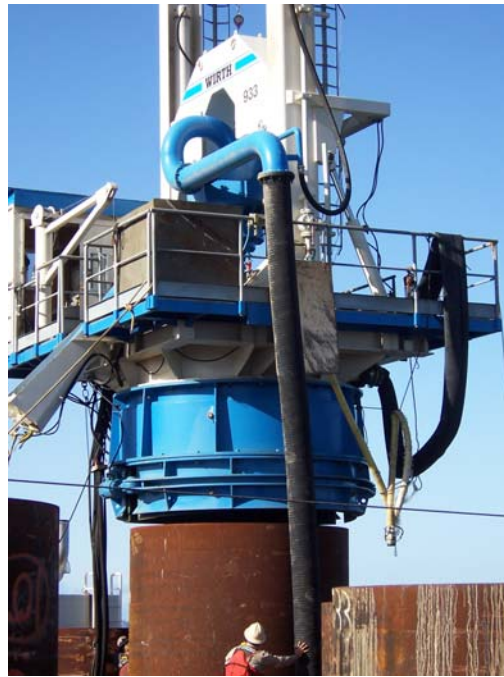
FIGURE 6-10 Reverse circulation drilling equipment
