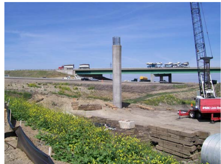
Bent 5 - side view of the column.
