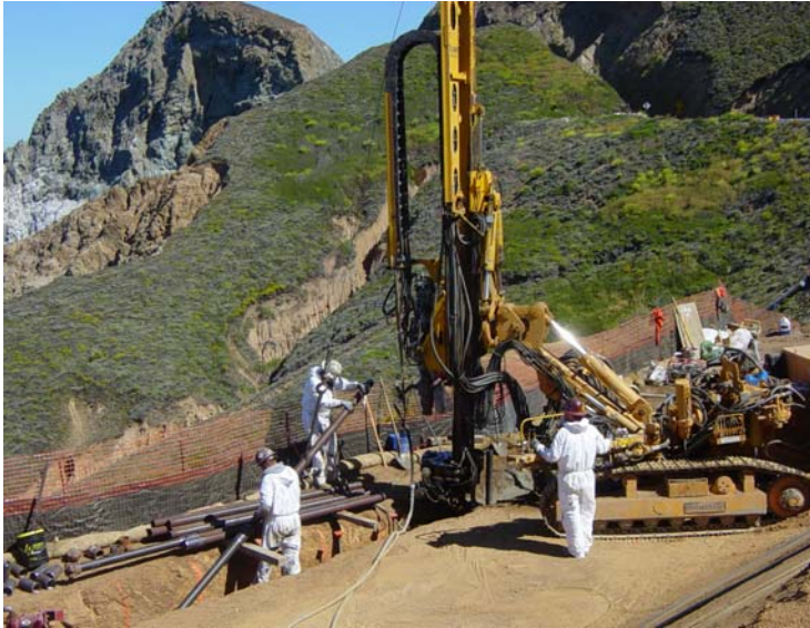
Lifting micropile pipe into place.
