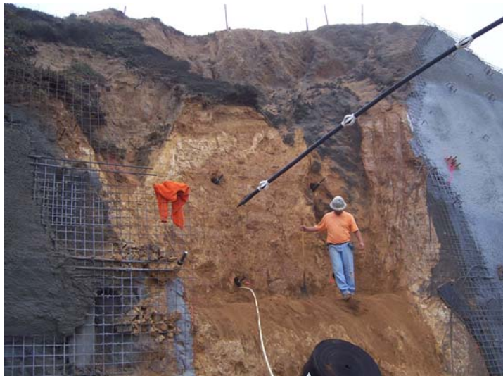
Soil nail getting ready to be installed in a drilled hole. Grouting lower nail w/1" PVC grout tube. 8/04/05
