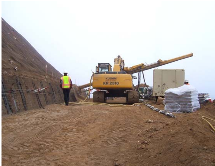
Drilltech drilling top row of nails at Wall #2. Test nail installed between two nails. 8/09/05
