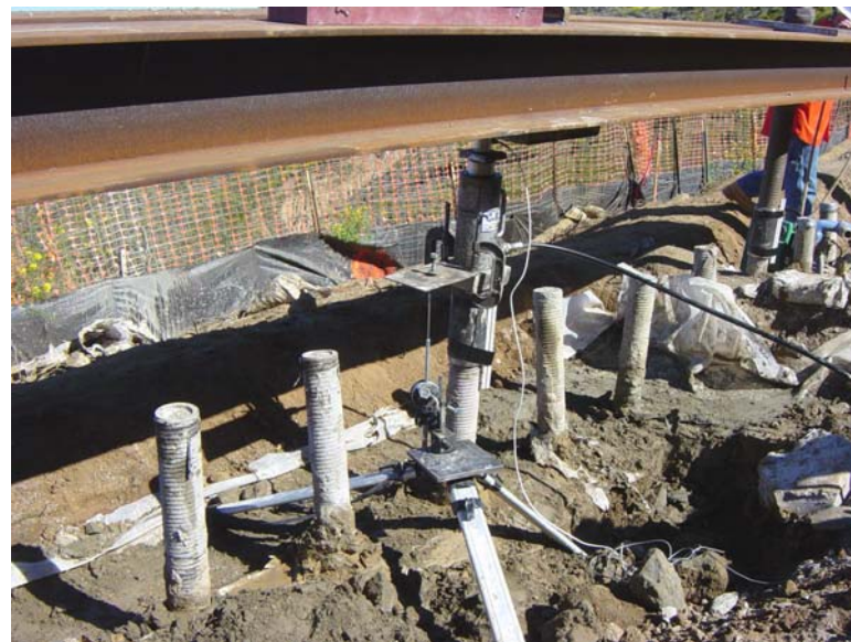
Hydraulic jack and measuring device.
