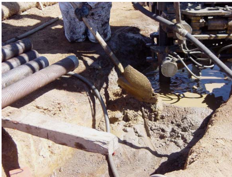
SWPPP: laborer is creating a check dam at each drill location to prevent grout and drill cuttings from covering next pile location.
