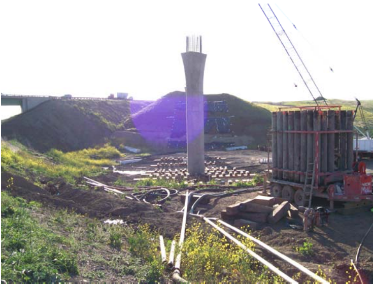
Bent 5 Column - After the forms were stripped.
