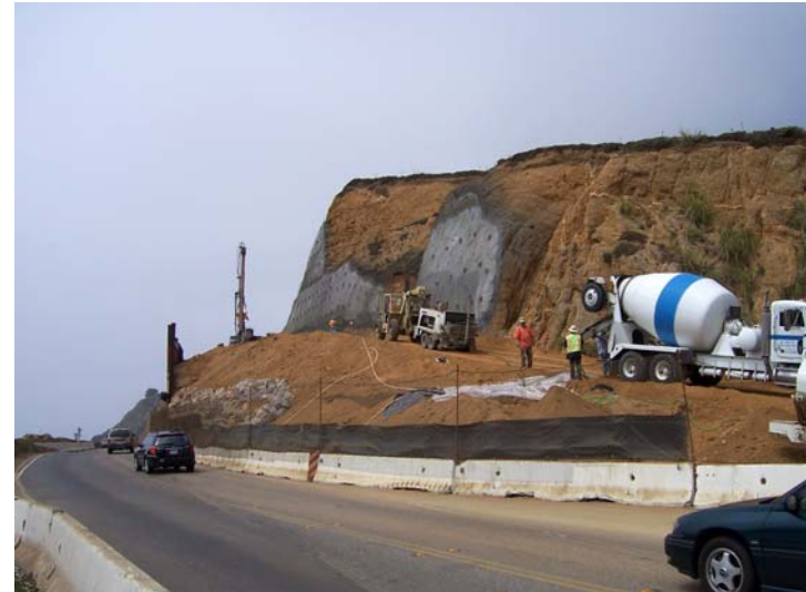
Drilltech shooting next section of initial shotcrete at Wall #1. 8/11/05
