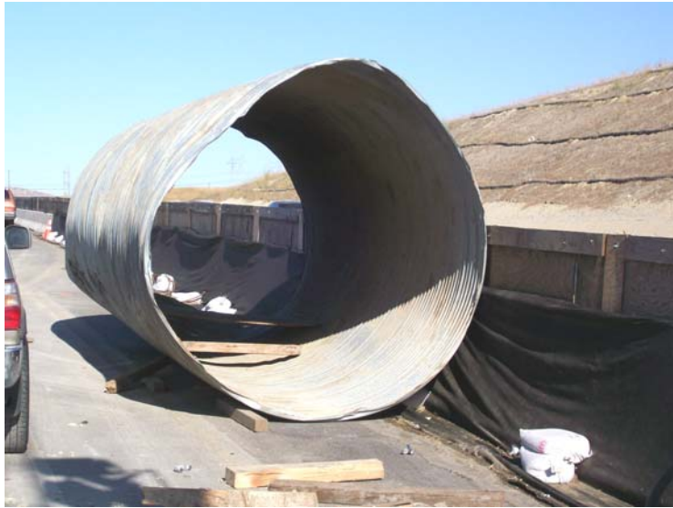
CMP casing used to prevent cave-in during drilling of the CIDH concrete piles.
