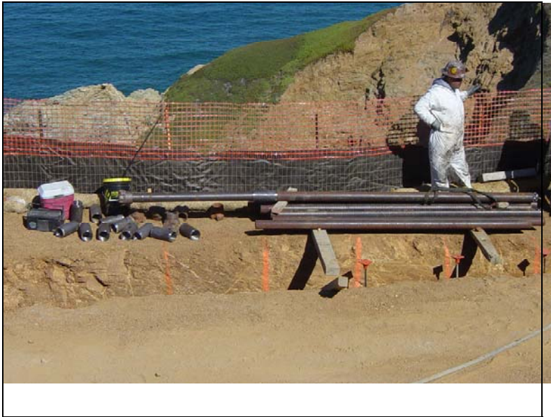
Assembled micropile components (Con-Tech Titan System): drill head, pipe (TITAN bar), pipe coupler.
