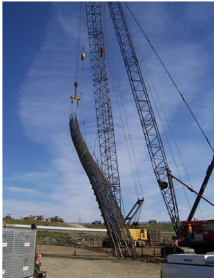
At the middle of the cage lift.
