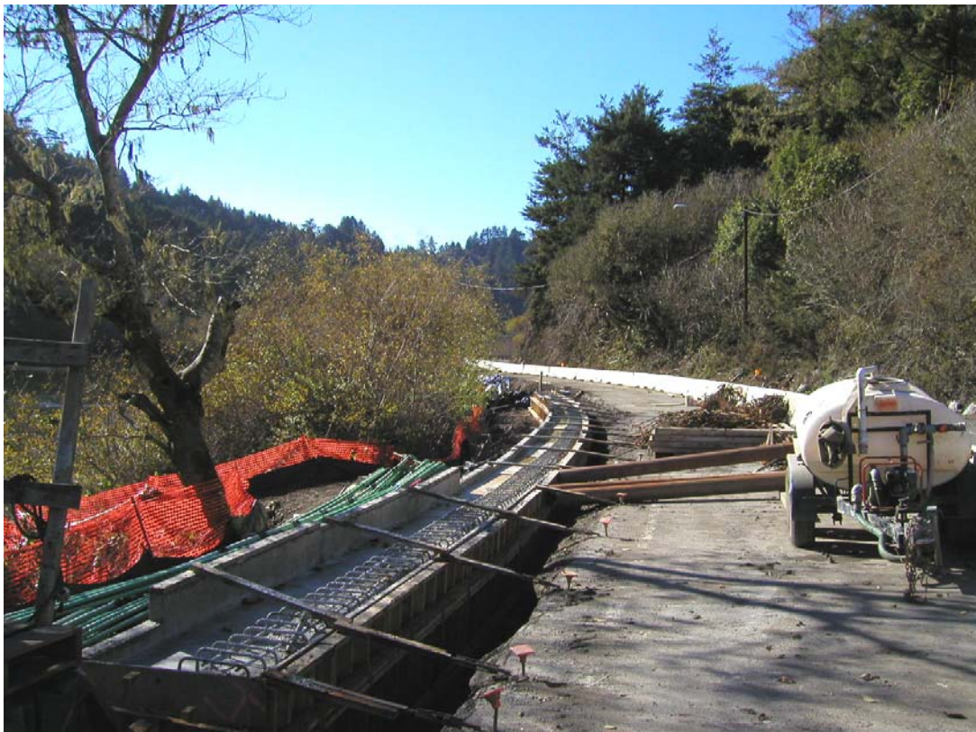
Cap beam construction.
