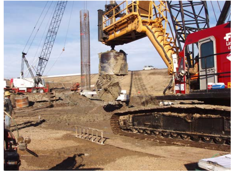
2.13-m diameter Clean out bucket cleaning out Bent 7 of the 580/205 Separation Bridge.
