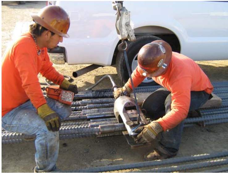
Iron Workers splicing the #43 rebar with BarGrip couplers.
