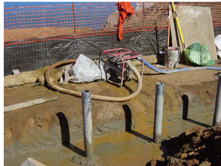
Portable pump used to pump excess grout and drill cuttings into settlement containers. Behind pump is silt fence and rolled straw.
