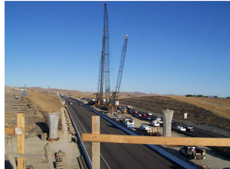
Vertical rebar cage lifted in the air.
