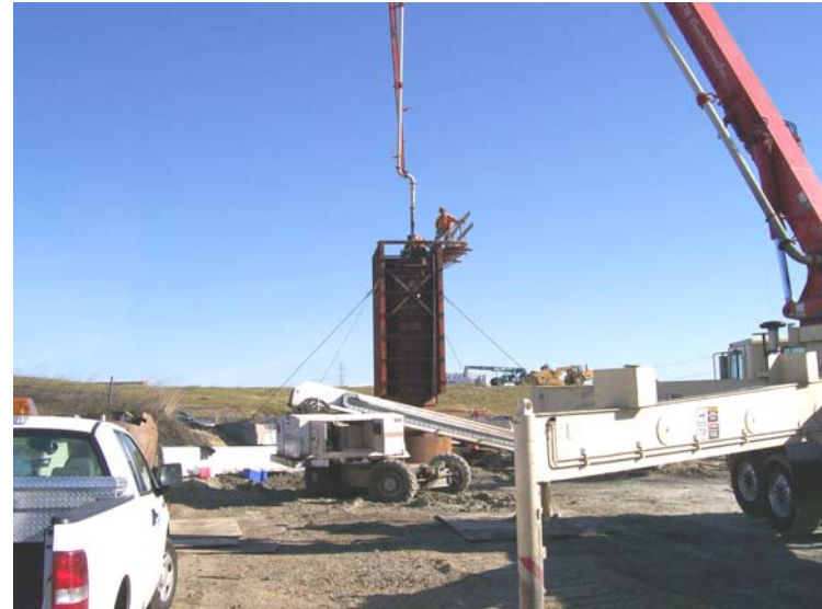
Guy wire in place during column pour.
