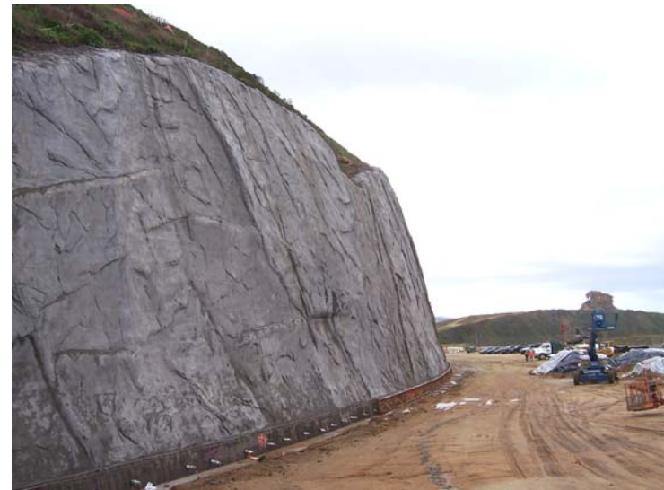
Type 60D barrier being installed at Wall #2. 03/21/06
