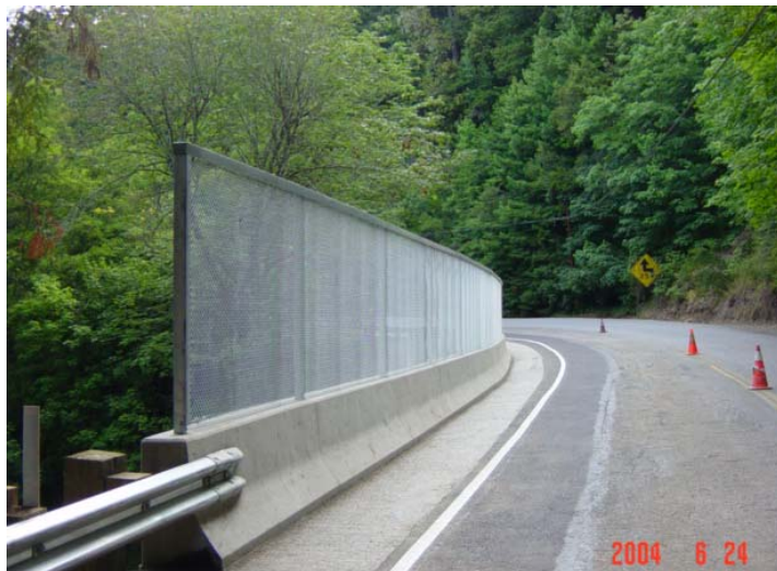
“After”. Facing east. Type 7 chain link fence. Type 27 modified concrete barrier on top of barrier slab. 6/24/04
