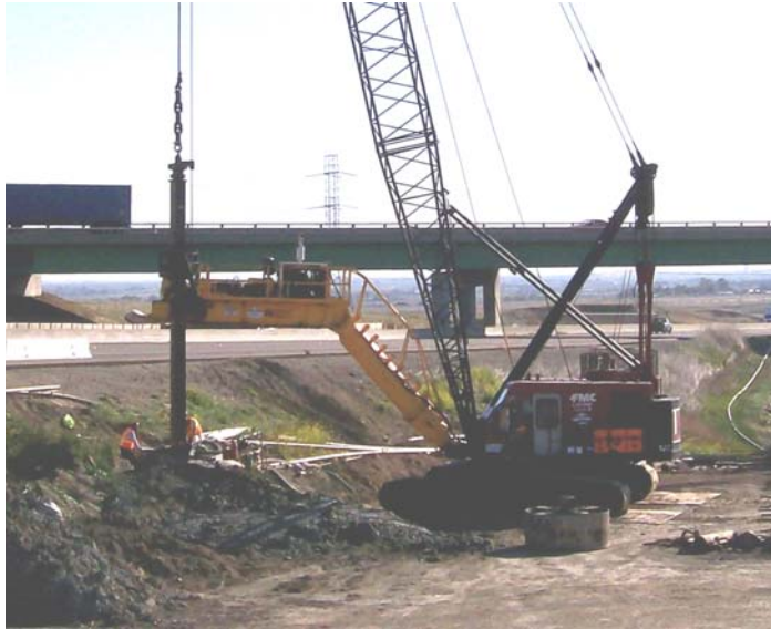
Link Belt LS-518 Crane with Steven M Hain Co 450K, Series 1 drill.
