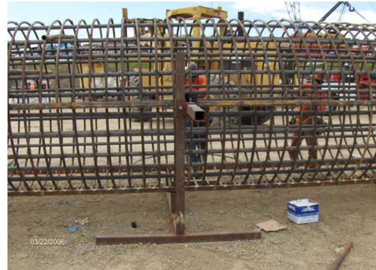
Iron Workers making the rebar cage at Bent 5.
