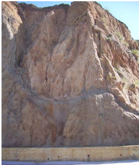
Southern end of Wall #1, after staining complete. Matches existing geology and color well. 04/18/06
