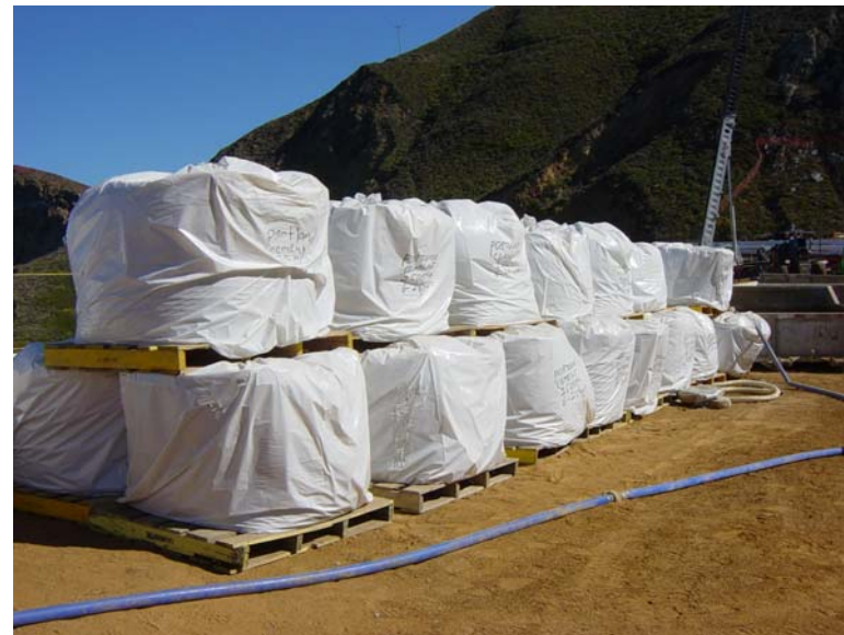
Cement sacks covered with plastic.
