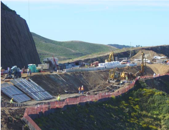
Site photo, facing south. South Rock Cut Retaining Wall (soil nail wall with sculptured face) on the upper left.
