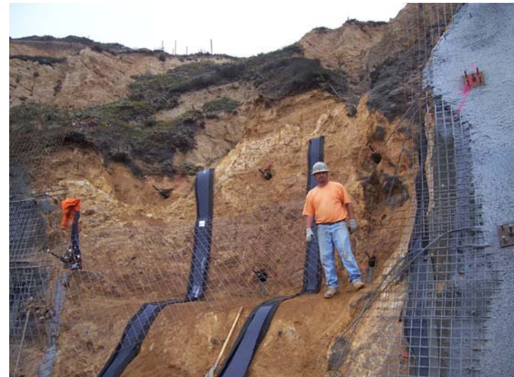
Drilltech crew installed 12" geocomposite drain strips between nail columns.
