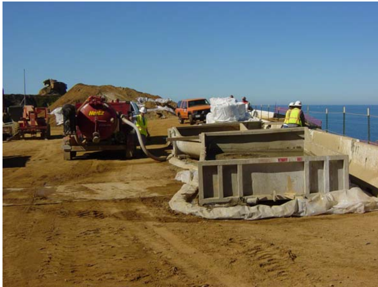
Storm Water Pollution Prevention Plan (SWPPP). Right: grout settlement container. Left: mobile tank and pump.
