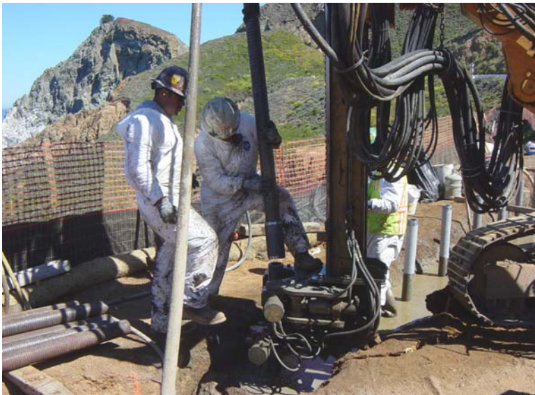
Adding another section of pipe (hollow treaded bar with coupler). Grout hose is in front of the man on the left.
