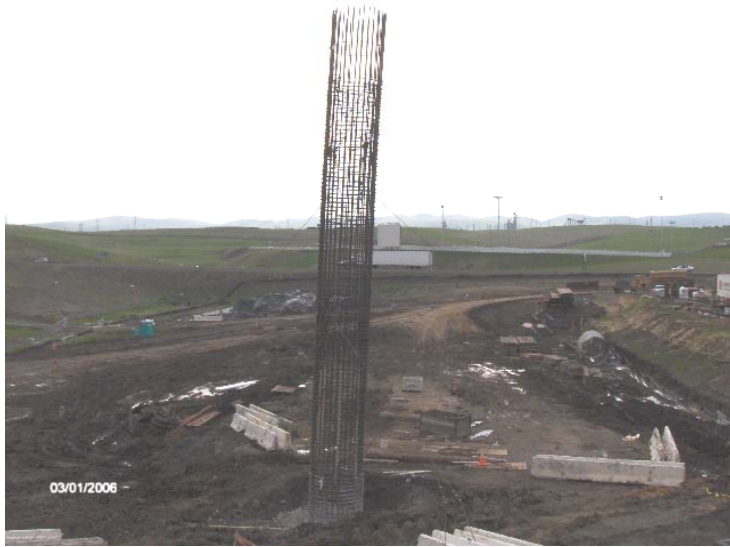
Guy wire placed near the top & middle of the rebar cage.
