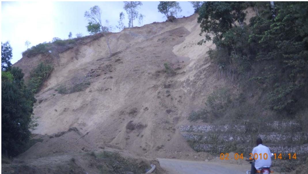
**Figure 9.11** Relatively shallow slip-out of regolith. Disaggregated material flowed over stable gabions and blocked over half the road. (N 18.409159, W72.638815).
