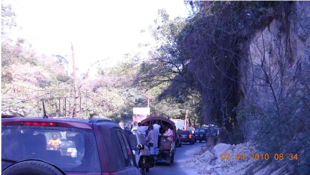
**Figure 9.5** Vertical cut remaining relatively stable with minor rock fall/topples.
