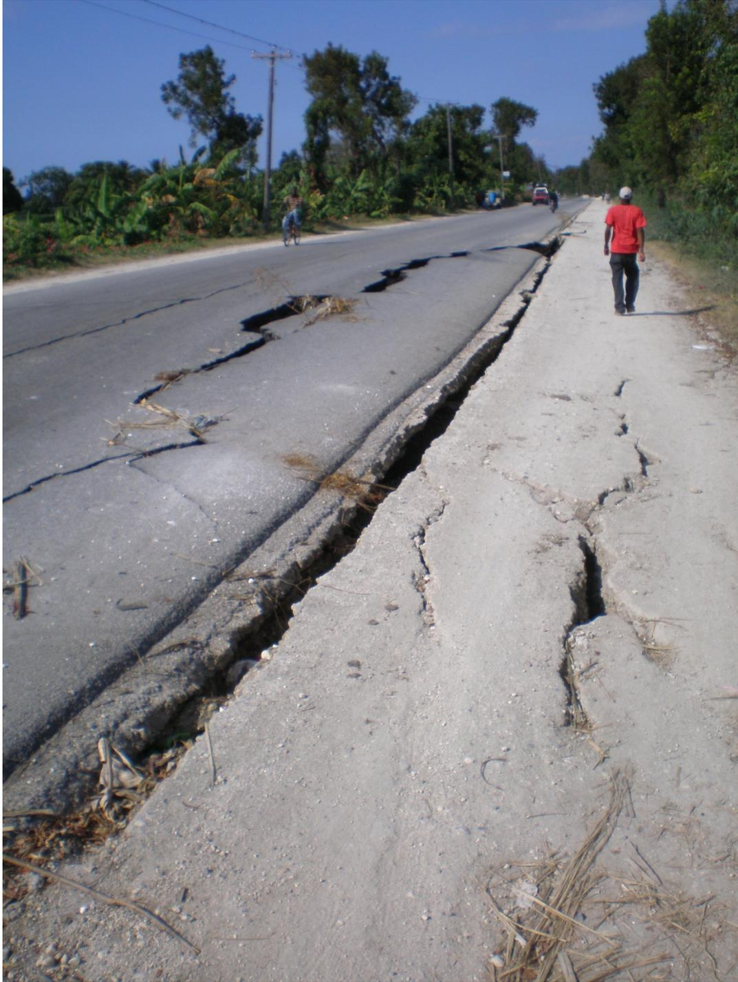
**Figure 8.5** Cracks induced by fill slope slumping at road damage site BOXCLVTA.
