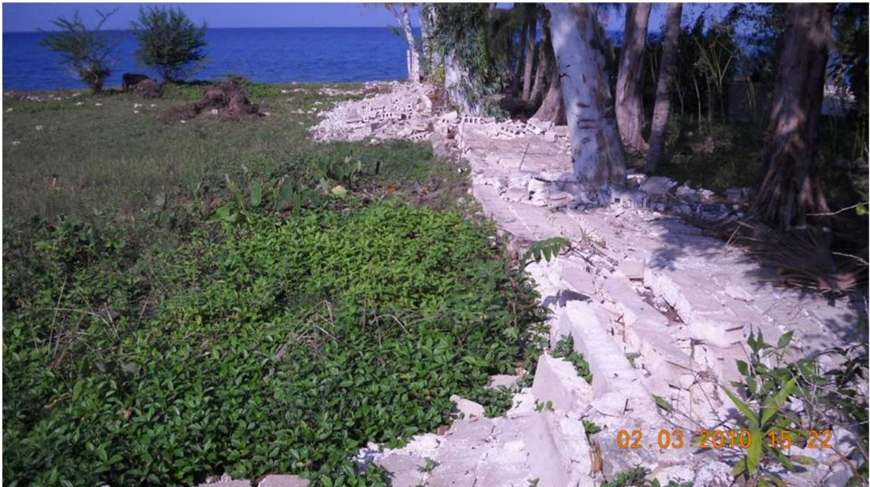
**Figure 7.20.** Damage to unreinforced block wall running perpendicular to coast near village of Grand Goâve. ( $18^{\circ}25'51.84''\text{N}$ ,  $72^{\circ}45'38.06''\text{W}$  looking northeast).
