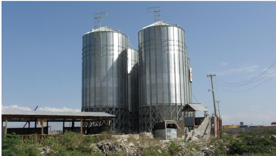
**Figure 6.19** Post-earthquake photo of steel grain hopper silos (photo taken facing North). The silos showed no visible signs of distress.
