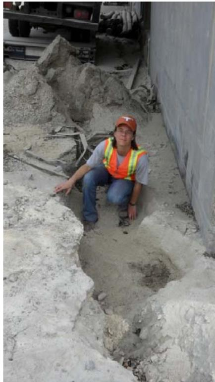
**Figure 6.10** Liquefaction and lateral spreading adjacent to the north side of the metal warehouses. Photo on top taken facing west, photo on bottom taken facing east. (N18.556961, W72.349751)
