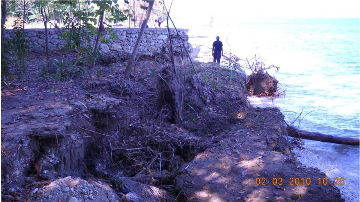
**Figure 7.11.** Damage to stone wall resulting from coastal failure and lateral spreading. (18°25'33.94"N, 72°43'34.27"W looking westward).
