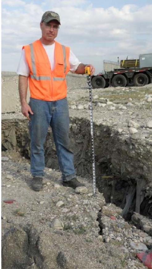
**Figure 6.24** Lateral spreading in the storage yards in the northern part of the port facility. A unique feature of this lateral spread is that the fill is garbage. However, it is believed that the liquefaction of the sand below garbage is the cause of the lateral spreading. Photo taken facing North-East. (Approximate long. and lat. of photo: 18°33'38.93"N 72°20'54.89"W)
