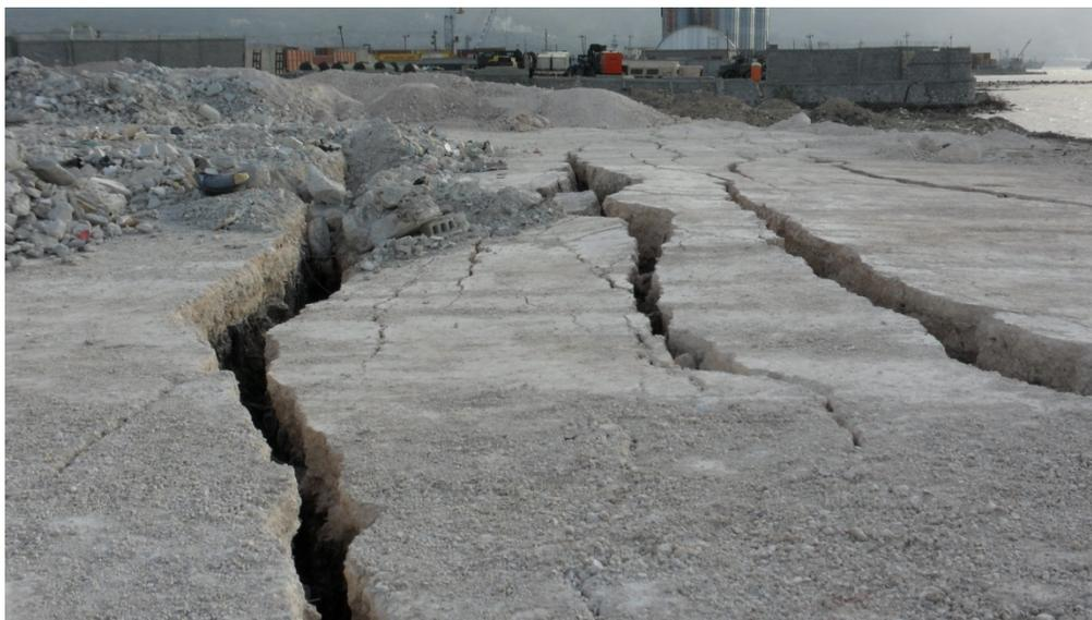
**Figure 6.21** Lateral spreading in the storage yards in the northern part of the port facility. Photo taken facing South. ( $18^{\circ}33'41.39''\text{N}$   $72^{\circ}20'52.51''\text{W}$ )
