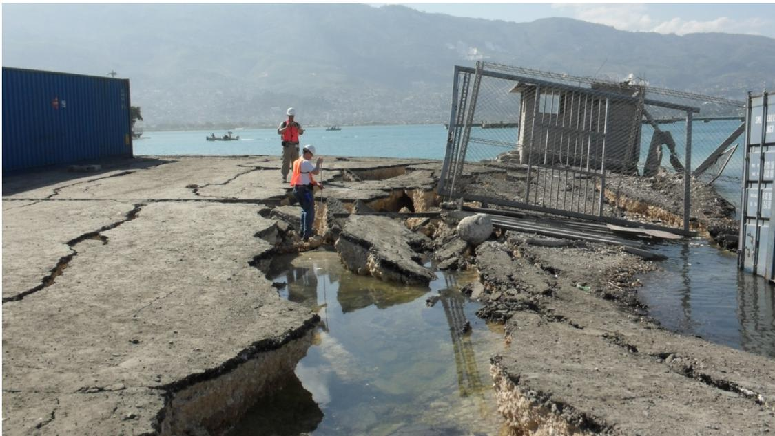
**Figure 6.9** Lateral spreading west of the two metal warehouses. Photo taken facing south with the metal warehouses to the left. (N18.557075, W72.352045)
