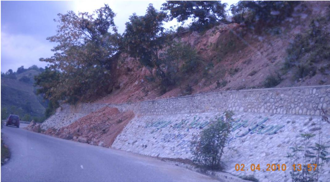
**Figure 9.12** Shallow slip-out of soil in upper road cut. Soil slid over the top of the surviving masonry wall and slope protection. (N18.440270, W72.636207).
