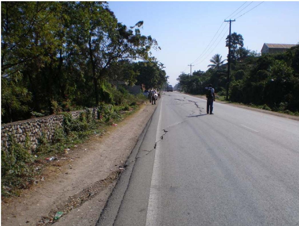
**Figure 8.4** Typical arcuate road cracks at road failure site RCA west of Carrefour.
