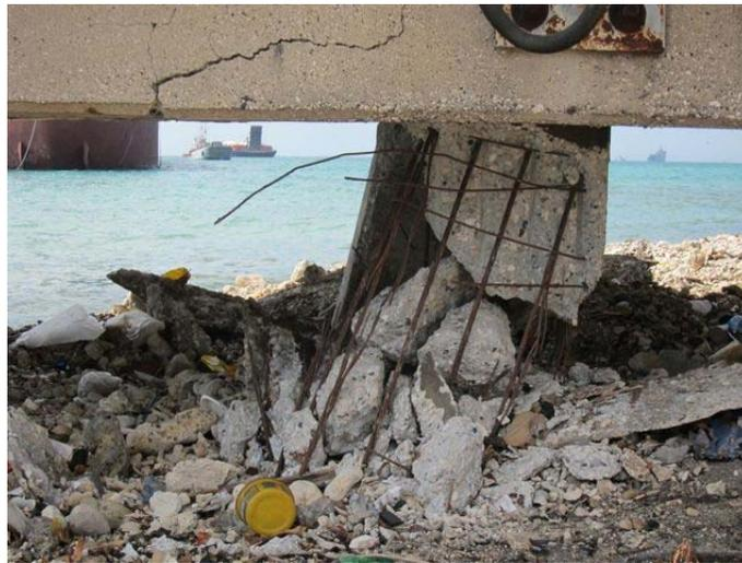
**Figure 6.16:** (top) Damage to piles supporting the pedestrian bridge connecting the South Pier to the island (photo taken facing South) and (bottom) extensive damage to the landward row of piles (photo taken facing West) (N18.554628, W72.351492)
