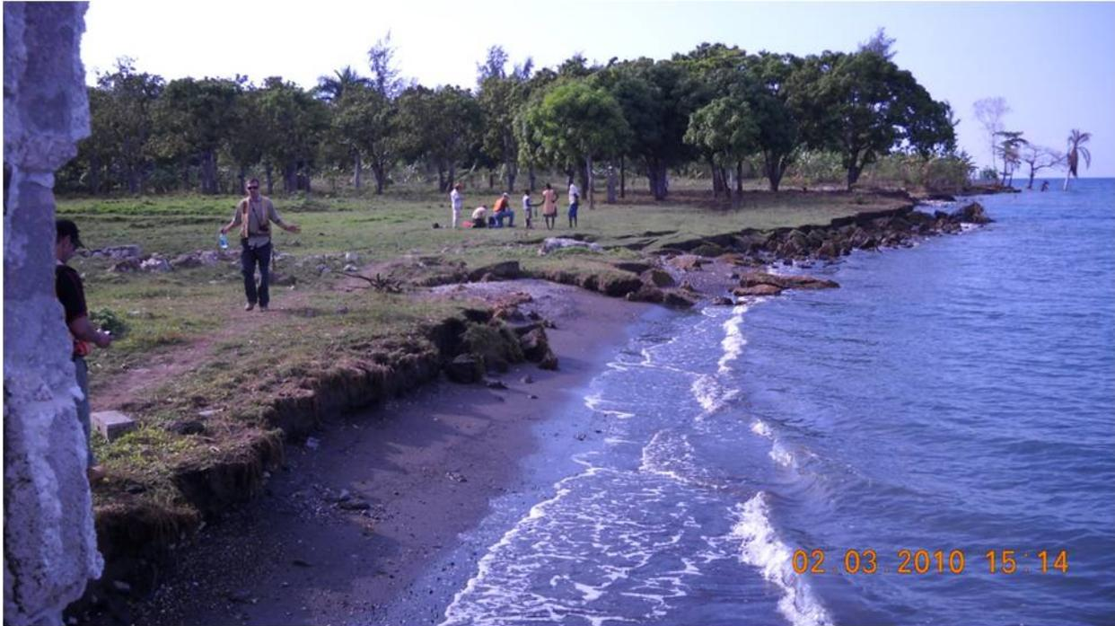
**Figure 7.17.** Scarp formed along northern portion of coastal failure near village of Grand Goave. ( $18^{\circ}25'53.82''\text{N}$ ,  $72^{\circ}45'37.16''\text{W}$  looking northwest).
