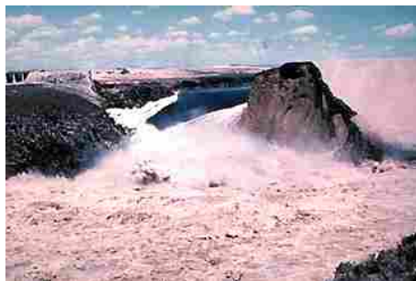
Figure 7.2: Failure of Teton Dam.
