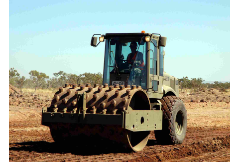
Figure 12.13: A road roller.
