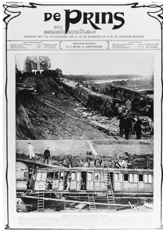
Figure 1.1: Landslide near Weesp, 1918.
