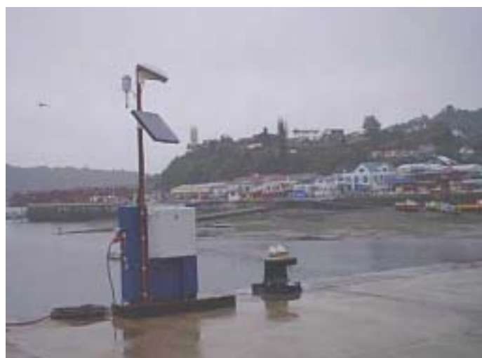
Picture of a Chilean Tide Gauge installed on a pier at Coquimbo bay (latitude 30° South) showing the water-proof case, the solar panel, the flat antenna and the pressure sensor.
