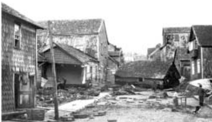
1960 Damaged caused by the May 22, 1960 Chilean Tsunami
