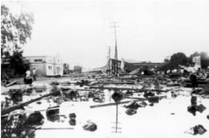
Destruction along the waterfront of Hilo, Hawaii from the Pacific-wide tsunami generated off the coast of Unimak Island, Aleutian, USA on April 1, 1946
