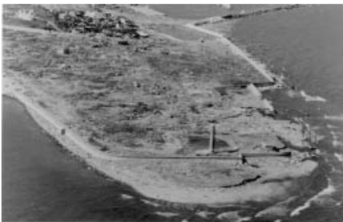
Massive destruction in the town of Aonae on Okushiri Island, Japan caused by the regional tsunami of July 12, 1993.
